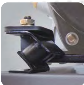
vibration absorber support the whole generator set
